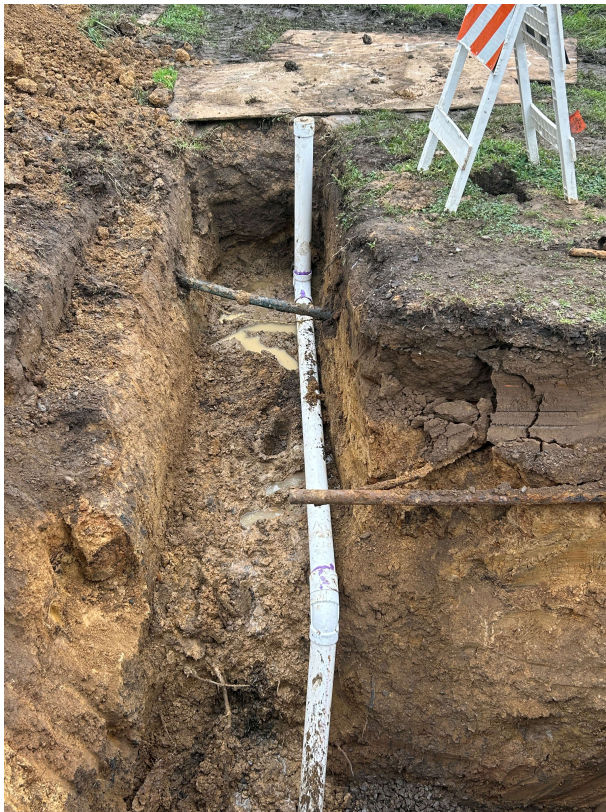
Lateral Service Line Installation
