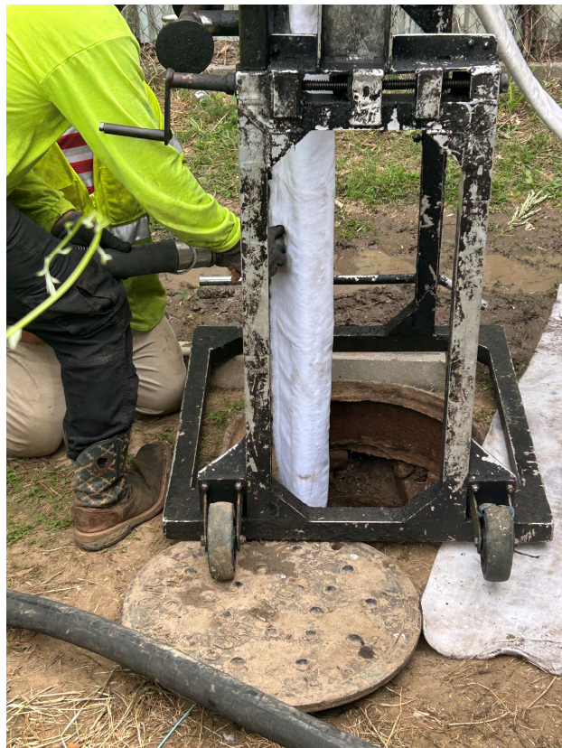
Installing Cured-In-Place Pipe (CIPP) Liner
