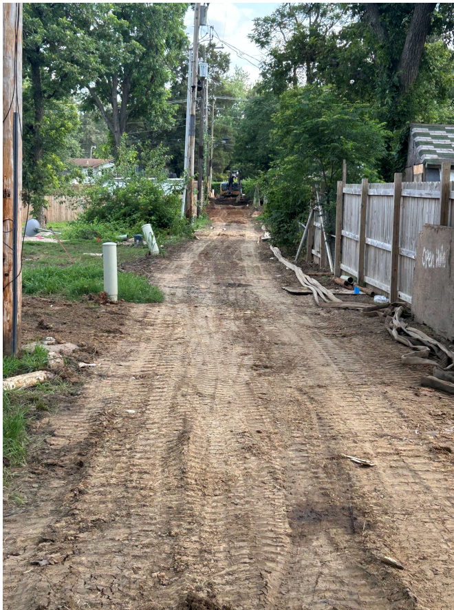
Alley Restoration Following Pipe Bursting
