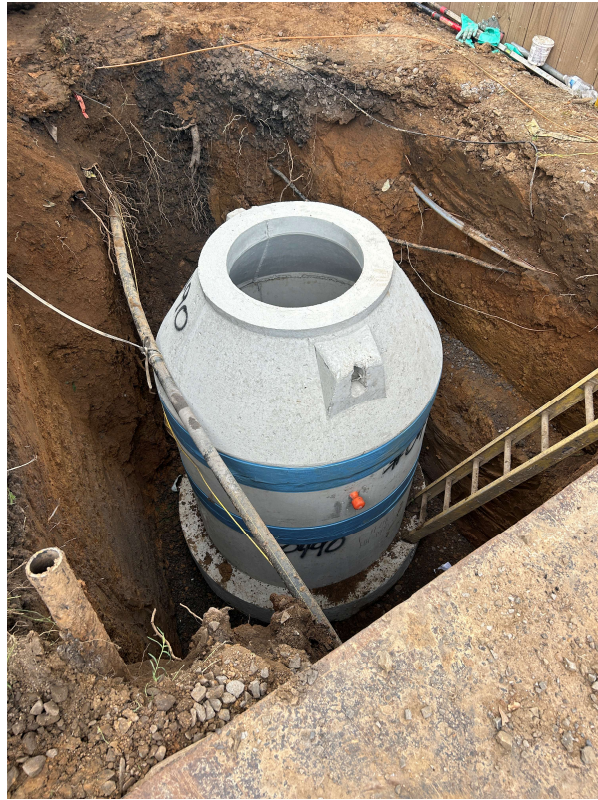
Installing New Manhole
